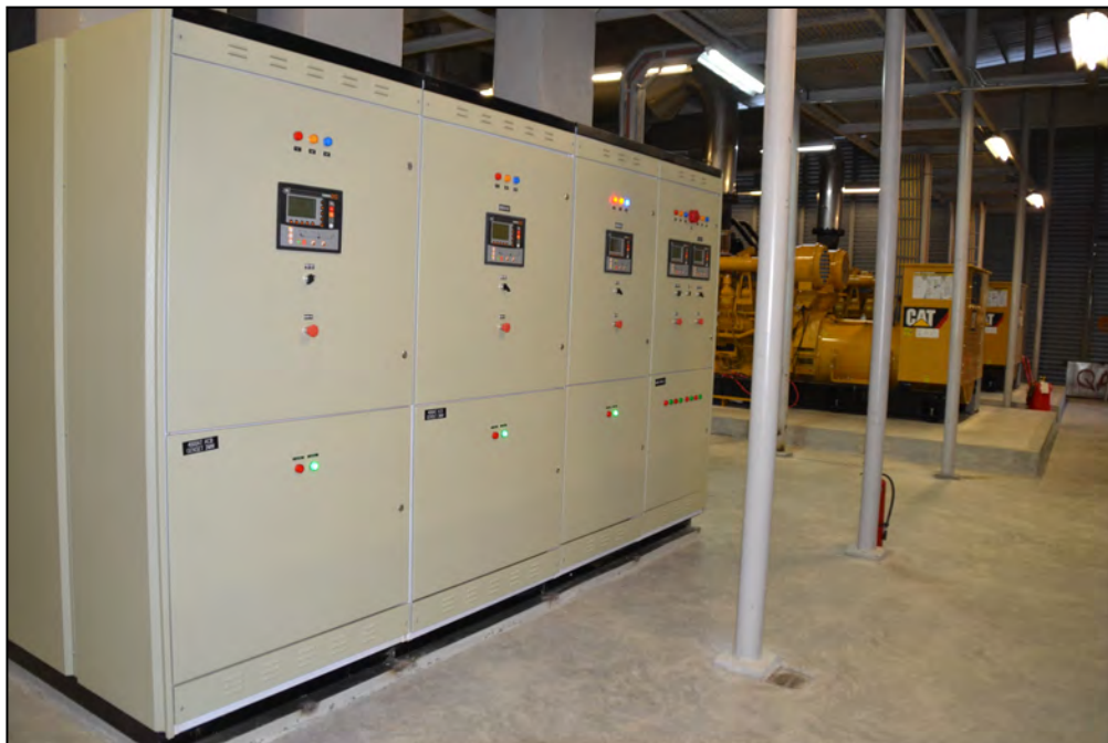
LV SOFT CLOSE TRANSITION ATS & SYNCHRONIZING PANEL for KCC MALL MARBEL, KORONADAL SOUTH COTABATO
