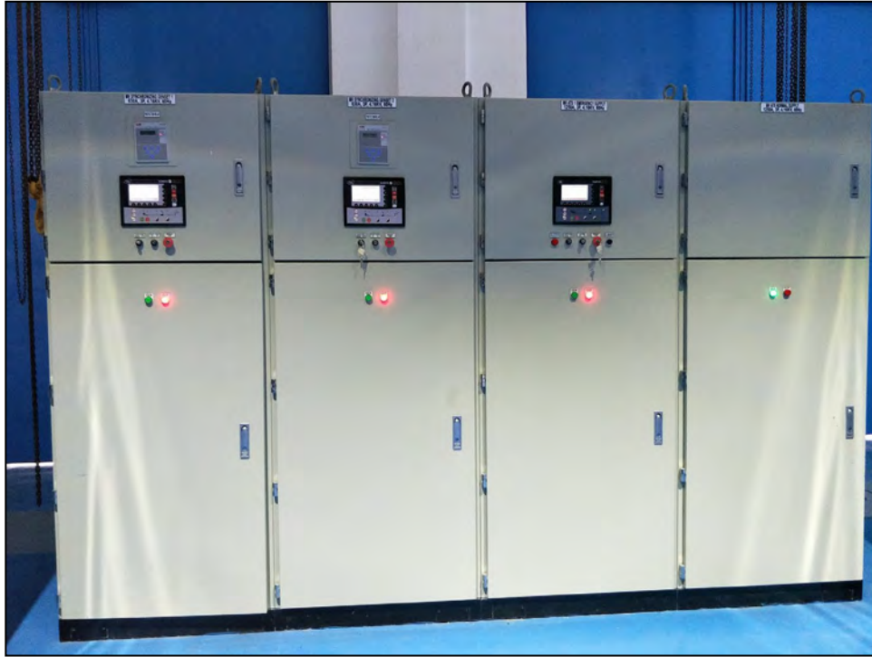
MV SOFT CLOSE TRANSITION ATS & SYNCHRONIZING PANEL for MAYNILAD LAMESA NORTH "A" ANNEX PS
