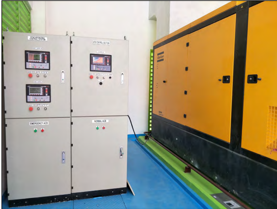
LV SOFT CLOSE TRANSITION ATS & SYNCHRONIZING PANEL for MAYNILAD MAGDIWANG PS & RESERVOIR
