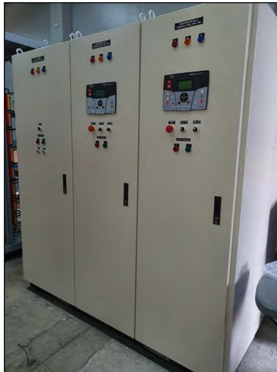
LV SYNCHRONIZING PANEL for TAGBILARAN IT HUB, BOHOL CITY
