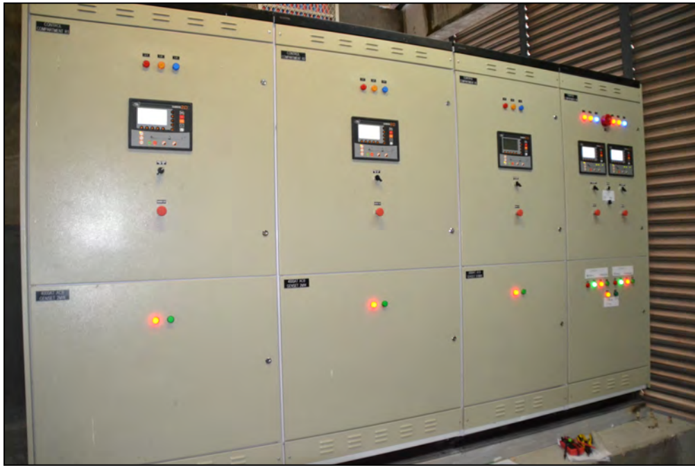
LV SOFT CLOSE TRANSITION ATS & SYNCHRONIZING PANEL for KCC MALL MARBEL, KORONADAL SOUTH COTABATO
